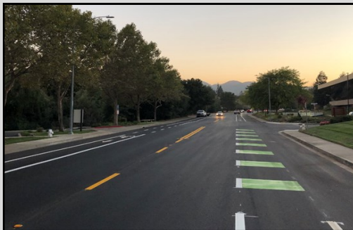
New Bike Lane—Old Crow Canyon Rd./Crow Canyon Rd.
