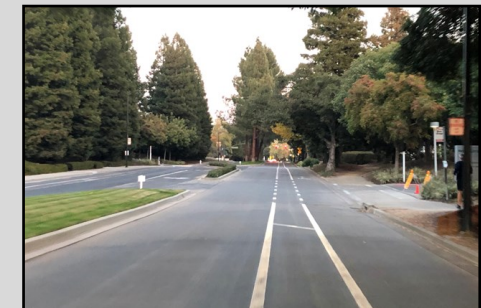
New Buffered Bike Lane—Executive Pkwy.
