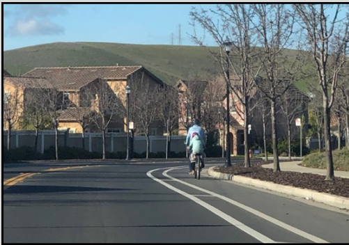
Buffered Bike Lane—Ivy Hill Wy.
